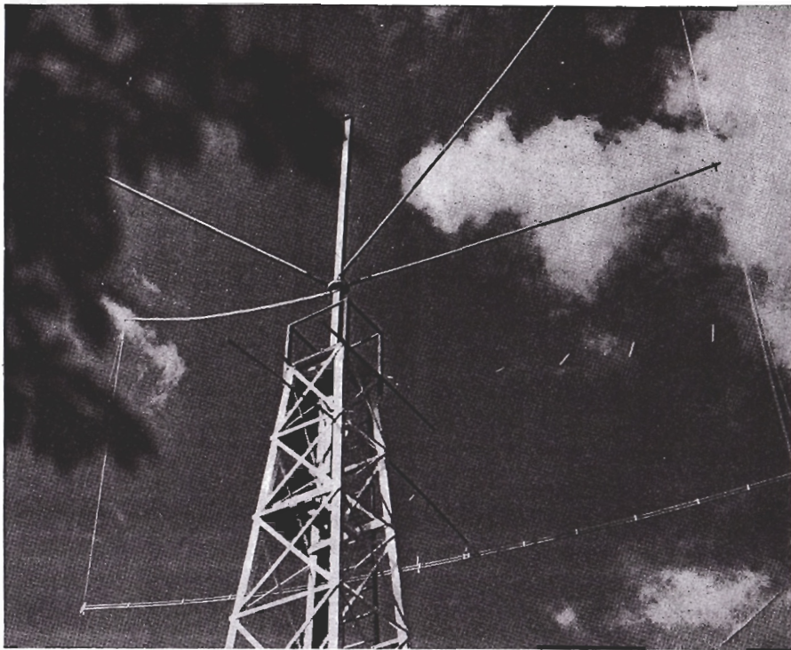
FIG. 80 — THE ISOLANTITE BLOCKS SHOWN IN FIG. 82 CAN BE SEEN PLAINLY IN THIS VIEW OF THE COMPLETED FOUR-ELEMENT ARRAY
